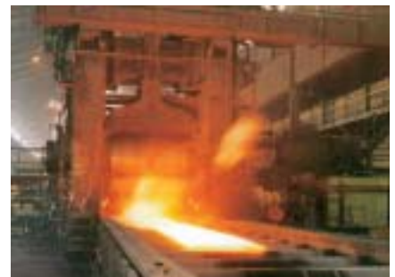
Rolling mill Galvanizing plant
